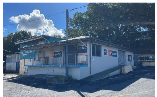
Figure 4 Building B Source: JBS&G
