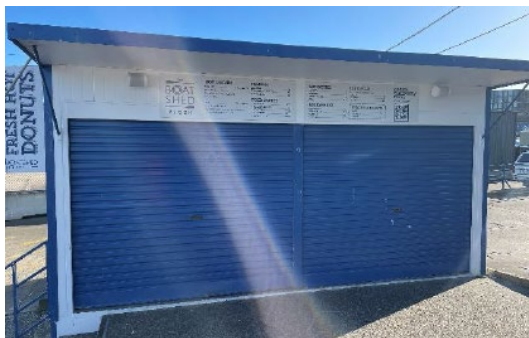
Figure 9 Kiosk Source: JBS&G
