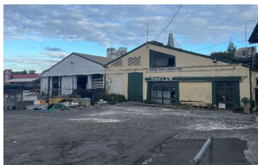
Figure 3 Building A Source: JBS&G
