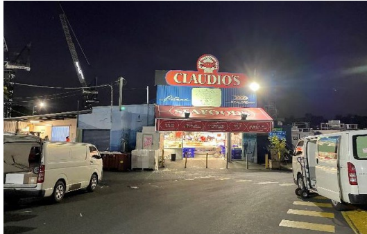
Figure 7 Building located north of Building D, previously occupied by Claudio's Seafood Source: JBS&G
